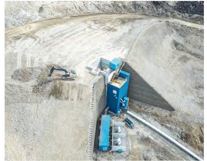
Primary Crusher MSE Wall – Over 26.5 m in height
