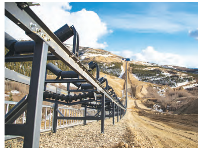
Overland Conveyor Earthworks
