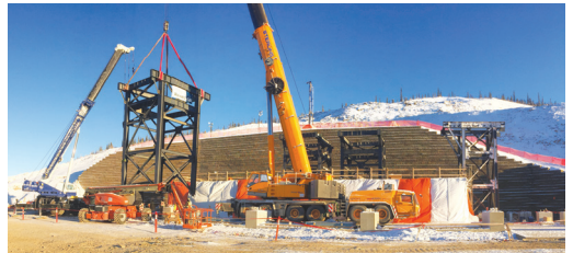
Hoisting steel at Secondary Crusher
