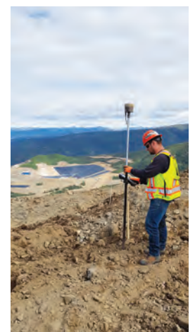
Eagle Gold Mine's road construction layout. June 2018.
