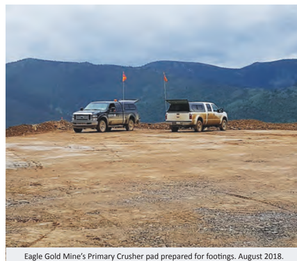
Eagle Gold Mine's Primary Crusher pad prepared for footings. August 2018.
